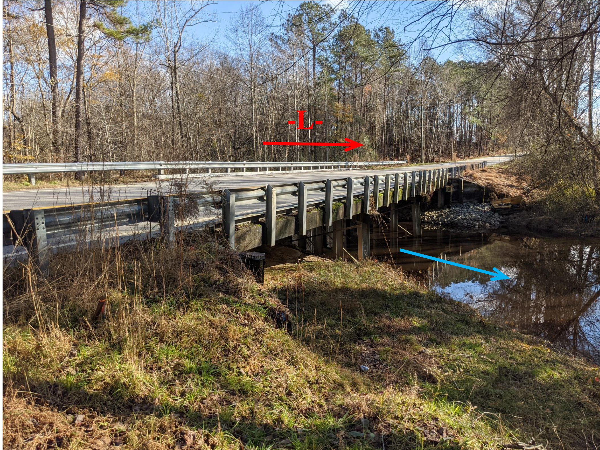
Looking South towards End Bent 2
